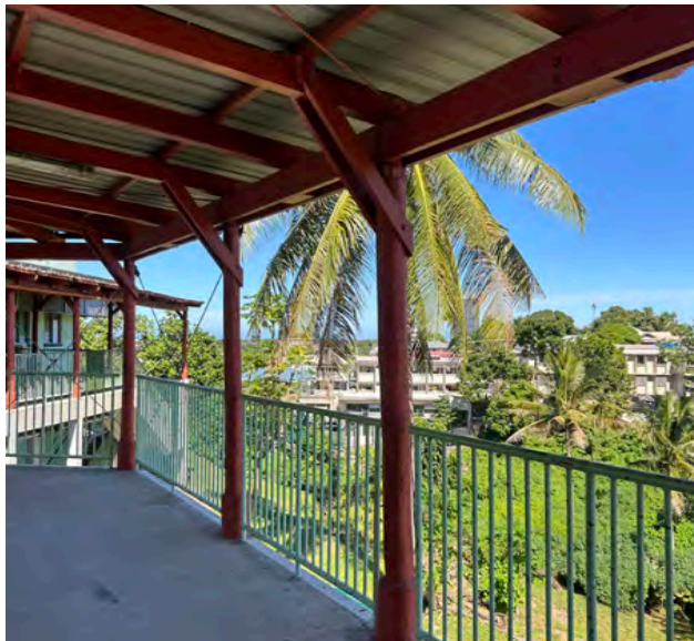
View from the corridor of the Colonial War Memorial Hospital when walking from the Paediatric Department to the operating theatres.
